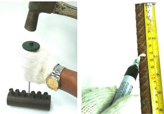
Mark the bar engagement length on each bar end, using the data in the table.
