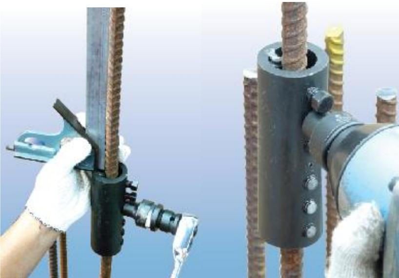
Insert the second bar into the coupler until contact with the centre pin and repeat the operation. Check the bar alignment when hand tightening the screws with a wrench : at a distance of 25cm the misalignment should not exceed 5mm (or not more than 1/4" at a distance of 1ft).
