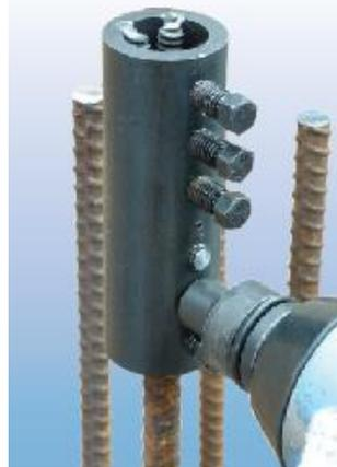
Tighten the screws, from centre to outside, with a power drive (pneumatic wrench) until their heads shear off. (A manual wrench can be sufficient for small screws – M12 & M16 – if there are not many couplers to assemble).
