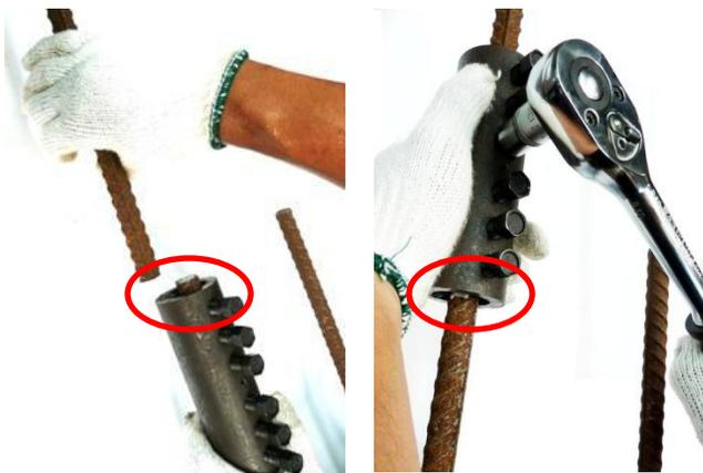
Slide the Unitec coupler all over the first bar. Bring the continuation bar in front of it and slide the Unitec coupler back over it. Position the coupler between the marks and hand tighten the screws.
