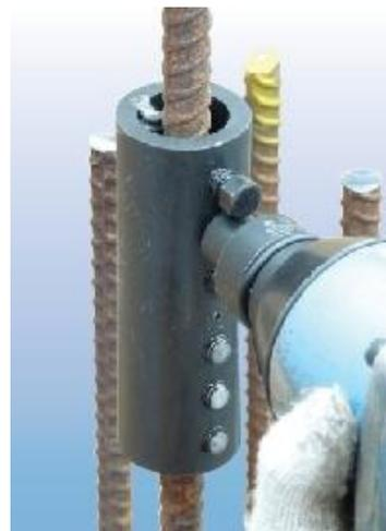
Tighten the screws, from centre to outside, with a power drive (pneumatic wrench) until their heads shear off.
