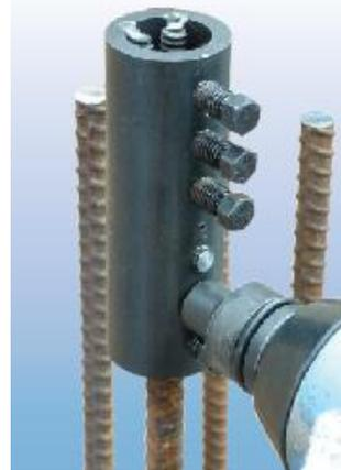
Tighten the screws, from centre to outside, with a power drive (pneumatic wrench) until their heads shear off. (A manual wrench can be sufficient for small screws – M12 & M16 – if there are not many couplers to assemble).
