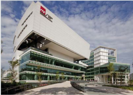
Ang Mo Kio ITE Headquarters, Singapore
