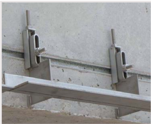
Brick work cladding fixed on anchor anchor channels
