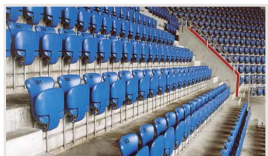
Stadium seating fixed on anchor channels
