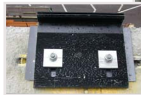
Curtain wall cladding fixed on anchor channels on the top of slab
